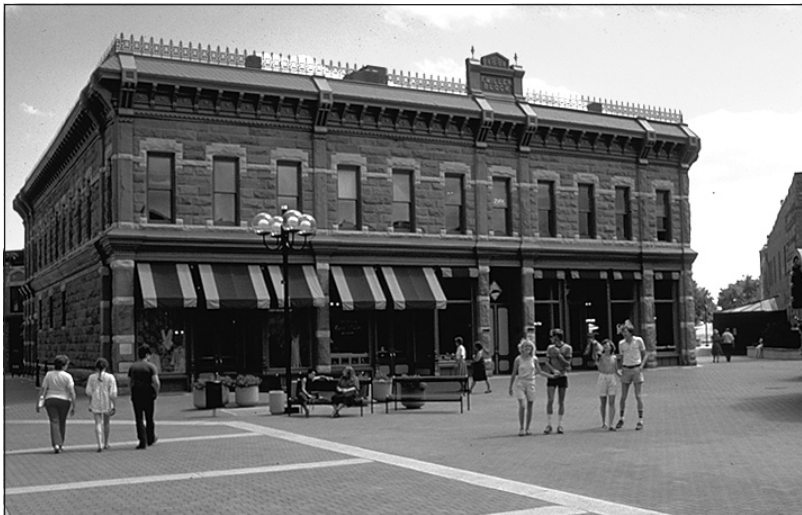
The Miller Block was restored, following Winter's Old Town Design Guidelines. The plaza in the foreground is a part of the Old Town Master Plan.
