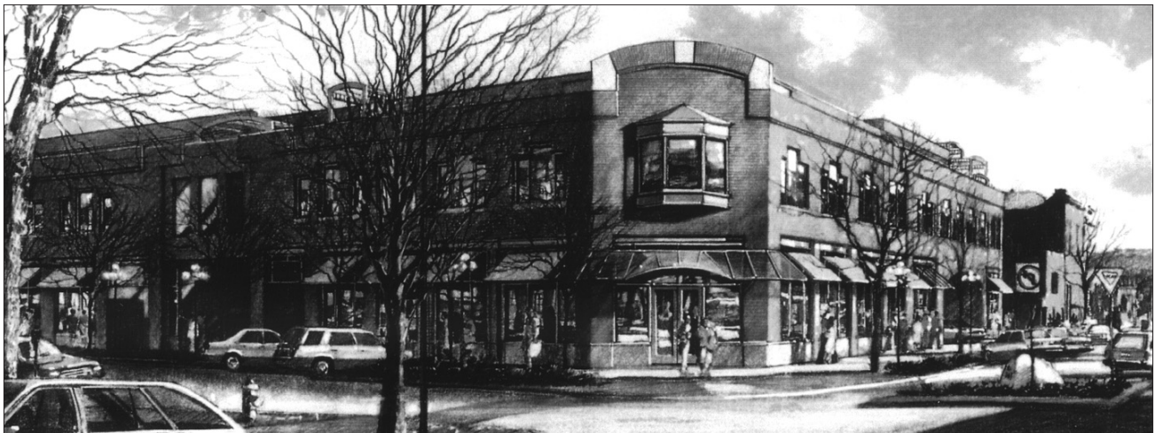
Design guidelines for downtown Boulder, Colorado, directed the developer of this parking garage to provide a two-story commercial storefront which relates to the traditional downtown character.
