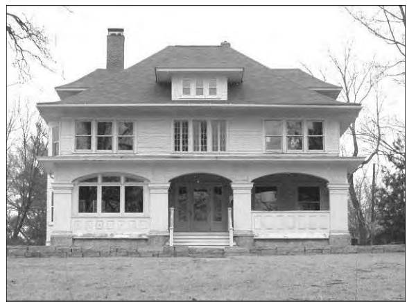
Large Foursquare house with Classic Revival details
