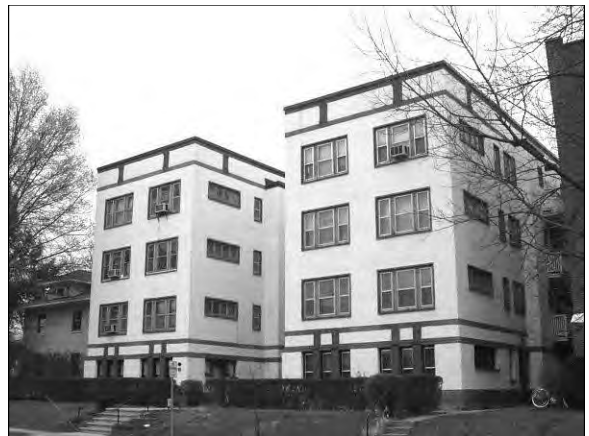
Stucco and brick Prairie School apartment building
