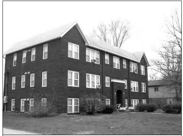
Vernacular apartment building with Period Revival influence
