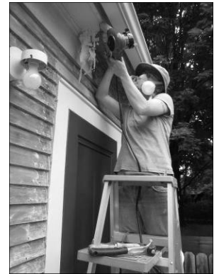
Proper usage of respiratory protection and heat to prevent the distribution of lead dust
