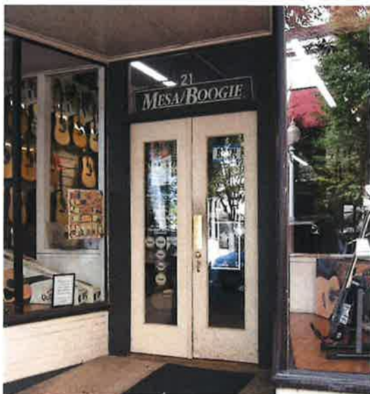
These historic single-light wooden doors above are an appropriate model for storefront doors.
