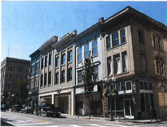
These two-part commercial blocks are consistent in design, with regular windows and sheet-metal cornices at the roofline.
