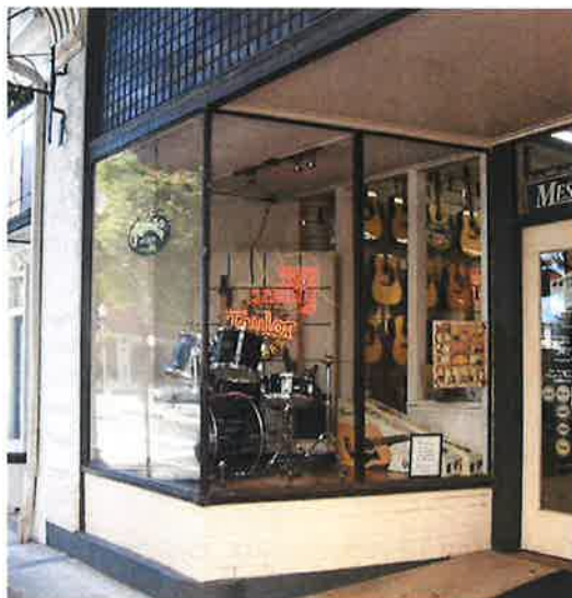
The large windows above are effectively used to advertise the business.
