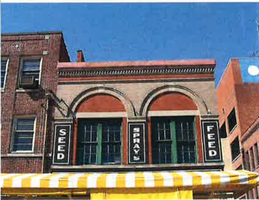
Masonry without serious mold, soot, or staining, should be maintained rather than cleaned.
