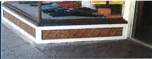
Several storefronts in the H-1 District have unique pressed-metal bulkheads; they should be preserved.
