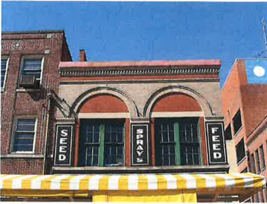
Upper-story windows are important in defining the architectural character of downtown Roanoke.
