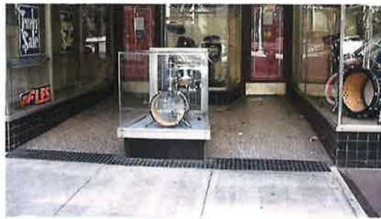
The different paving used in this recessed entry distinguishes it from the adjacent sidewalk, as was historically typical.
