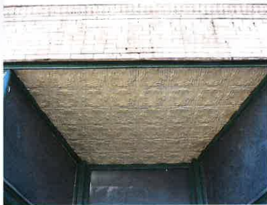
Maintain historic ceiling materials.
