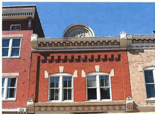
This building displays brick corbelling and a sheet metal cornice.
